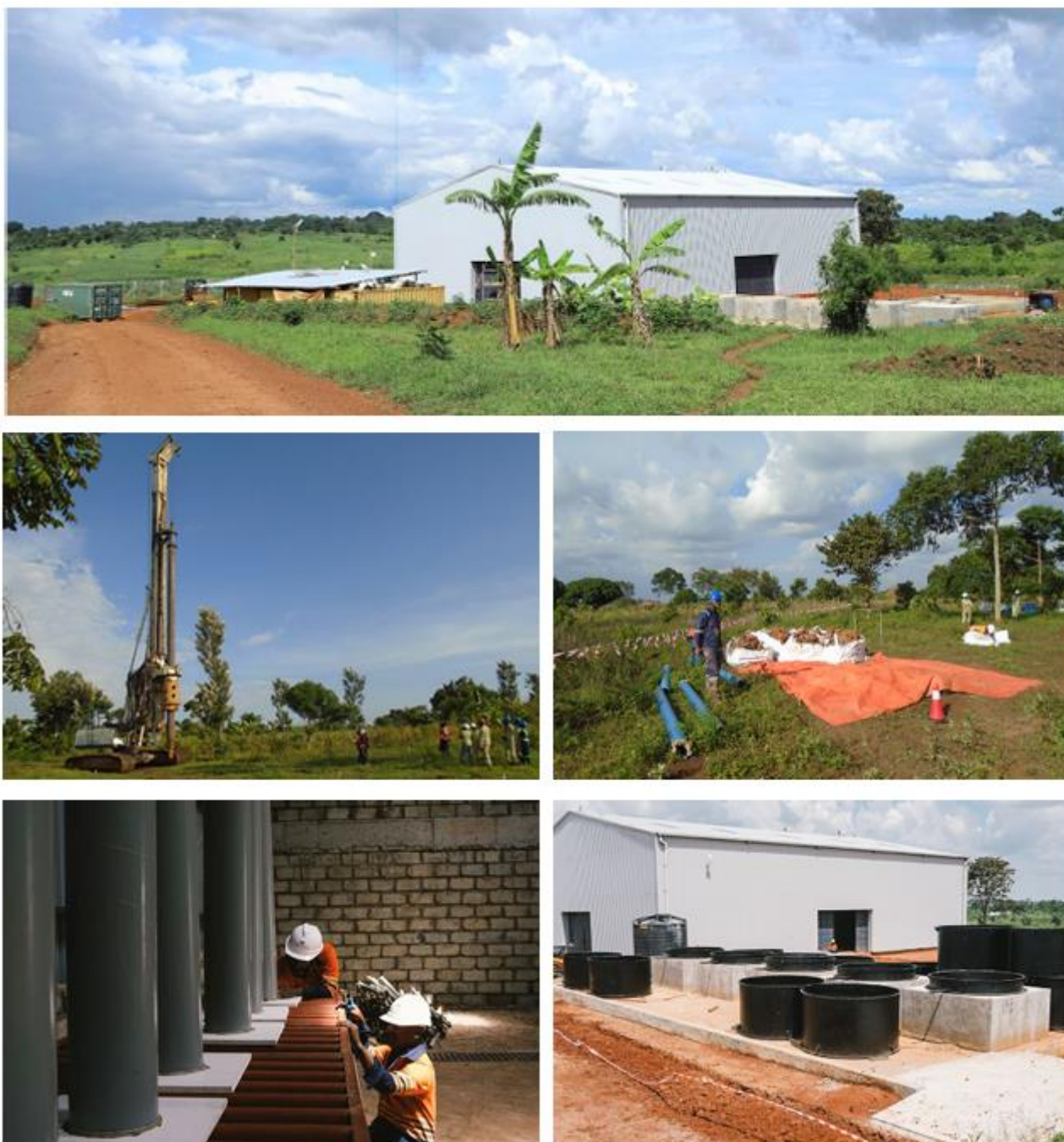
Figure 6: Makuutu Demonstration Plant nearing completion on site in Uganda
