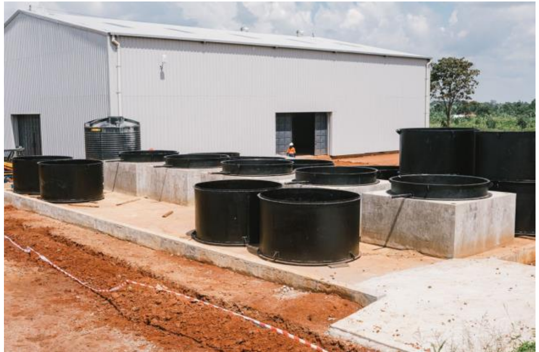
Figure 5: Demonstration plant nearing completion
