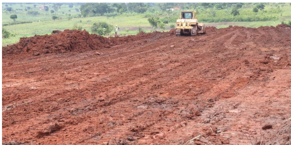
Figure 3: Demonstration plant earthworks progressing
