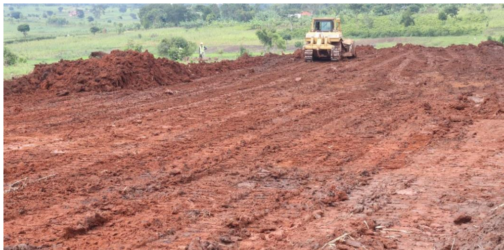
Figure 3: Demonstration plant earthworks progressing
